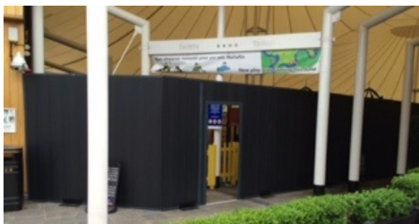
Left: An indoor hoarding creates a works compound within a garden centre at McArthur Glen, Bridgend, Wales.
