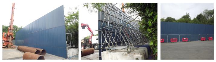
Our Ultraspan system was supported by a steel scaffold and concrete block matrix, creating a 6m hoarding
