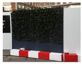
Trays of water are placed behind the Ultraspan hoarding to feed the ivy roots during dry weather
