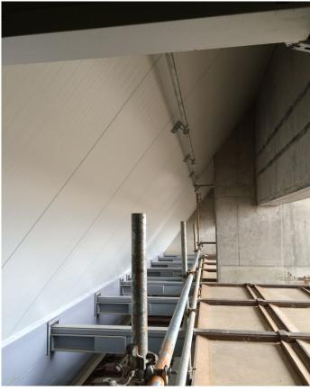
6m high panels were cut to size and sealed to provide an angled dust screen
