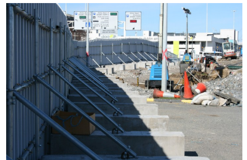
A high security robust hoarding is established
