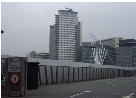
A view from inside the extensive 810m perimeter and vehicular entry gates—also made from recycled plastic
