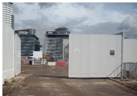
A view from inside the extensive 810m perimeter and vehicular entry gates—also made from recycled plastic
