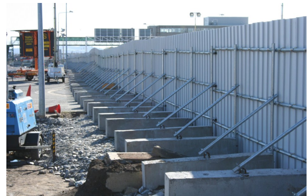
A high security robust hoarding is established
