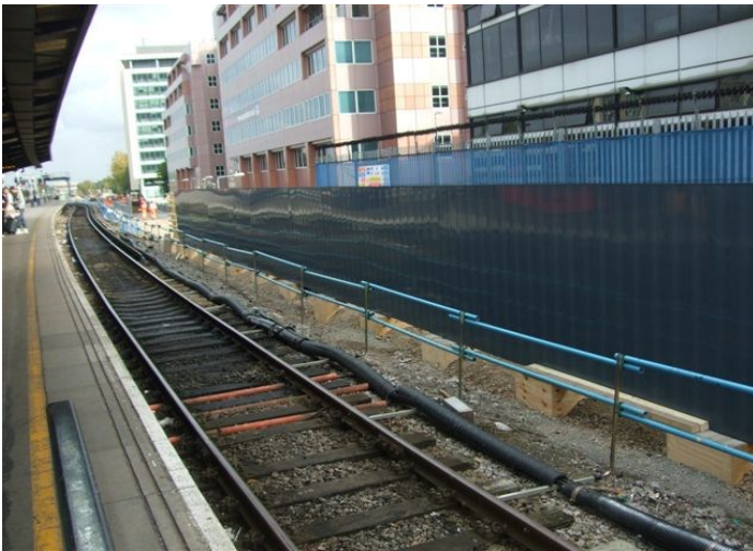
View from platform 4 of the finished hoarding.
