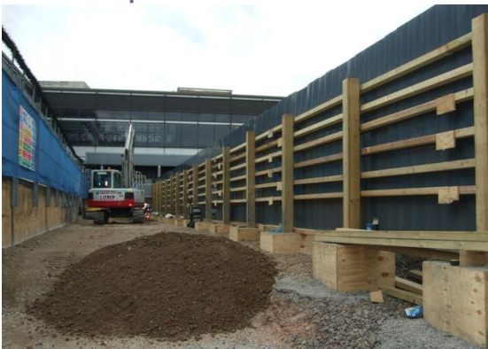
Network Rail R-11 specified Hoarding Systems with timber frame facilitates piling works near Platform 4.
