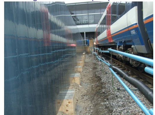
Network Rail R-11 specified Hoarding Systems with timber frame facilitates piling works near Platform 4.
