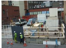
Vehicular gates are created with Ultraspan panels on a steel frame. Timber frames are used for the perimeter.
